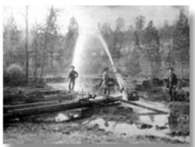
Hydraulic mining for gold, with water monitors to wash away the ancient river channels. Near Mountain Ranch in 1880
